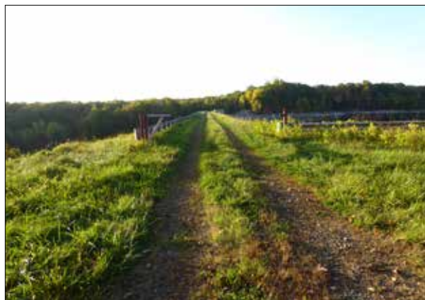
Upper Trinity Lake Reservoir Dam Pamela Corey
