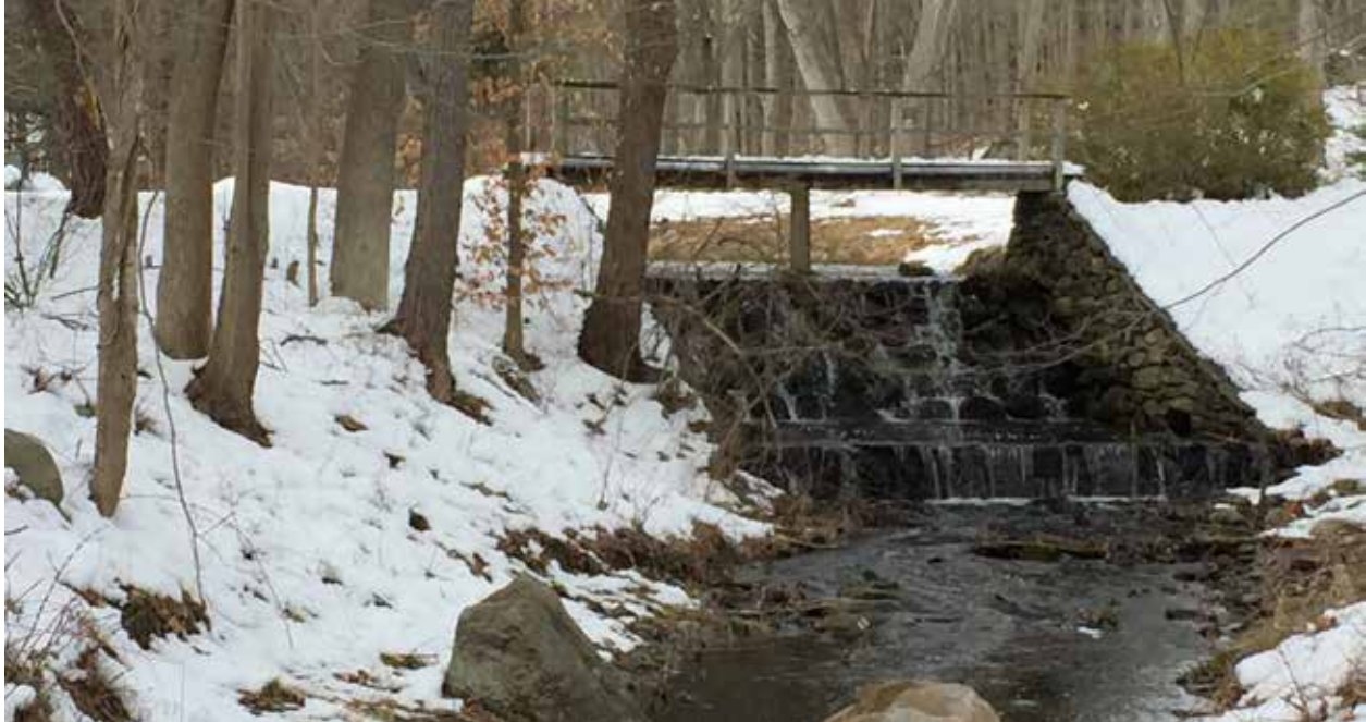
H.J.Halle Dam on Salem Road C. Reppert 2018
