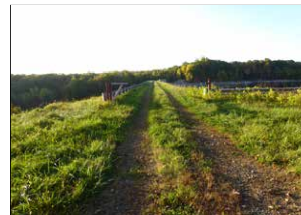
Upper Trinity Lake Reservoir Dam Pamela Corey
