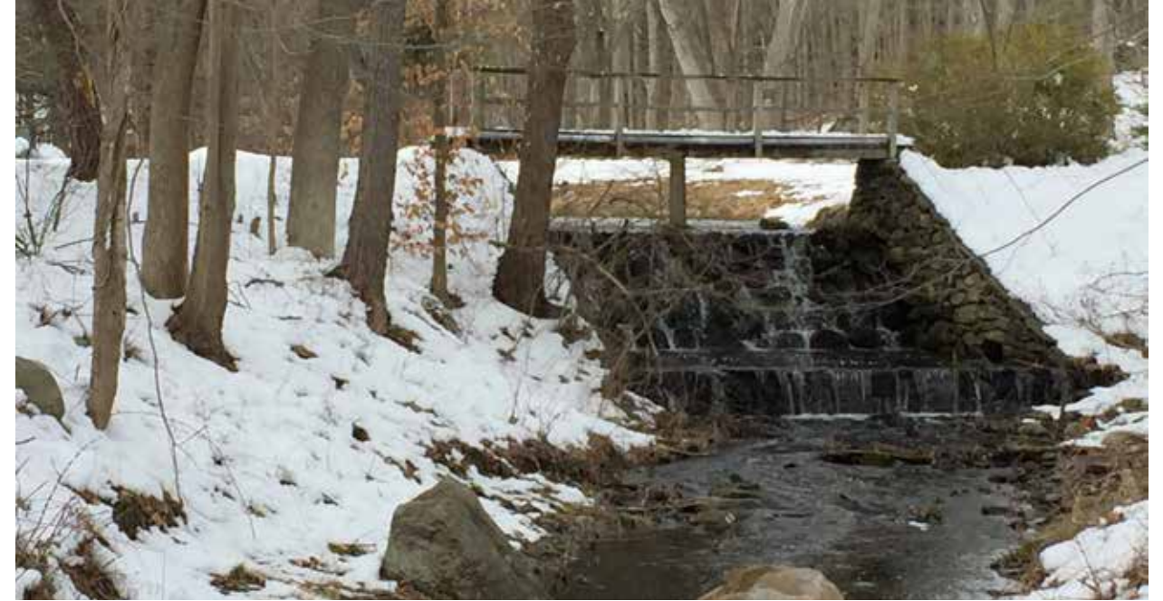
H.J.Halle Dam on Salem Road C. Reppert 2018
