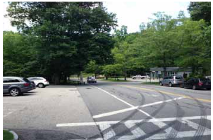
Western Approach South Of Roadway Lacks Sidewalk Or Enhancement To Alert Motorists Pedestrians Exist
