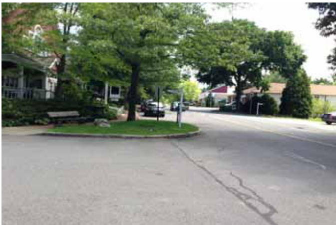
Existing Sidewalk North Of Roadway Ends About 400' East Of Town Trail
