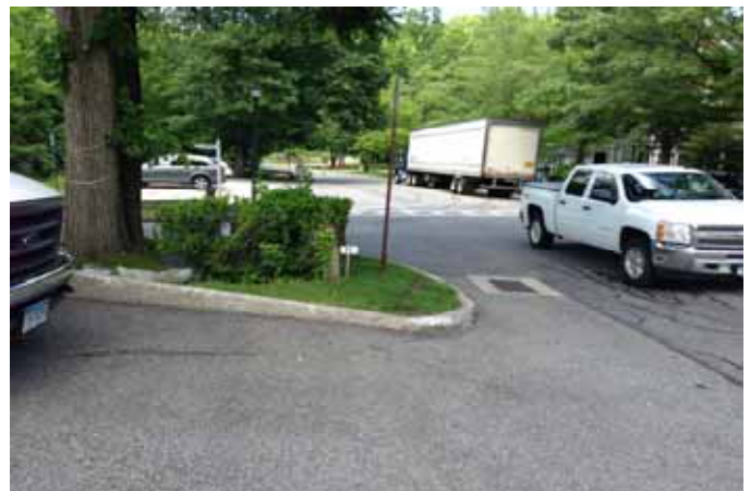
Some Curb Extensions Exist Without Pedestrian Provisions.
