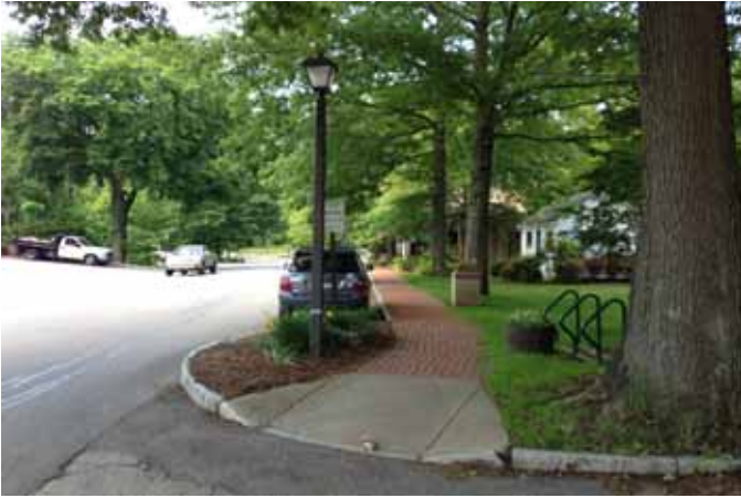
Curb Extensions Exist But Do Not Provide A Uniform Travelway Width. This Random & Overly Wide Width Contributes To Speeding And Bicycle Conflicts
