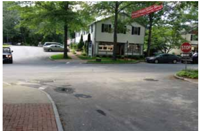
Crosswalks Are Not Well Defined Or Well Positioned
