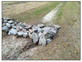
Check dams (if present): water is flowing around the edges of check dams, creating erosion or sinkholes on the uphill or downhill side, or the check dams are breaking apart or breaching.
