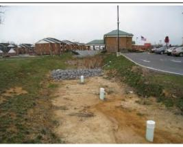
There is erosion on the surface; water seems to be carving out rills as it flows across the filter surface, or sinkholes are forming in certain areas.
