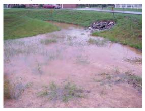
Water is still visible on the surface and/or the standpipe (if present) more than 72 hours after a rainstorm. The filter practice drains very slowly or is completely clogged.
