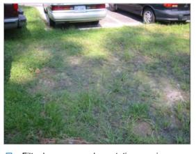
☐ Filter has grass and vegetation growing on more than 25% of the filter bed, threatening to clog the filter.
