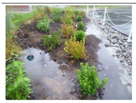
The bottom of the Bioretention cell is not flat, and the water pools at one end, along an edge, or in certain pockets. The whole bottom is not uniformly covered with water. See design plan to verify that bioretention surface is intended to be flat. Check during or immediately after a rainstorm.
