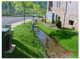
Water stands on the surface more than 72 hours after a rainstorm and /or wetland-type vegetation is present. The Bioretention cell does not appear to be draining properly. ☐ Kick-Out to Level 2 Inspection: This is generally a serious problem, and it will be necessary to activate a Level 2 Inspection.
